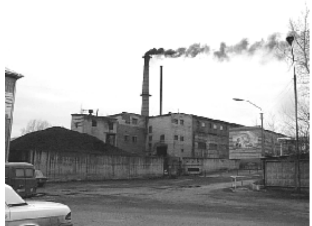
Fig. 2. Smoke plume of the PFCI boiler plant.
